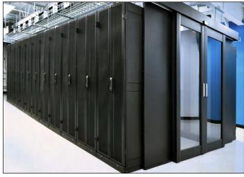
The doors of the CAC were a critical component to pressurize and seal the environment.
