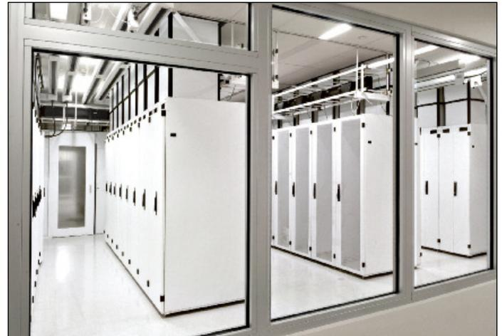
In an effort to build the greenest colocation facility in Oregon, the BendBroadband Vault deployed CPI Passive Cooling® and heat isolation by installing the F-Series TeraFrame® Cabinet System with Vertical Exhaust Ducts.
