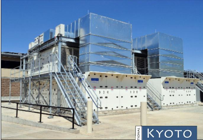
Two of the largest KyotoCooling® wheels in North America were installed at the Vault. Combined with CPI cabinets, they offer free cooling and a PUE as low as 1.2.
