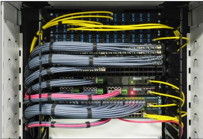
CPI’s Finger Cable Manager accessory and Vertical Cable Manager with T-shaped cable guides have cable openings that align with each U space for patch cord management.
