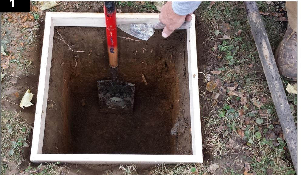
Dig a hole at least 16" x 16" minimum in the desired location for the assembly. The hole depth is determined by the frostline of the installation location. 30" is the minimum recommended. The sidewalls must be flush and plumb. Uneven sidewalls can cause the foundation to fail or tilt.
