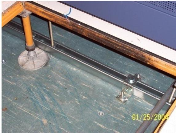
Fig. 2.2.1 Subfloor bracing
