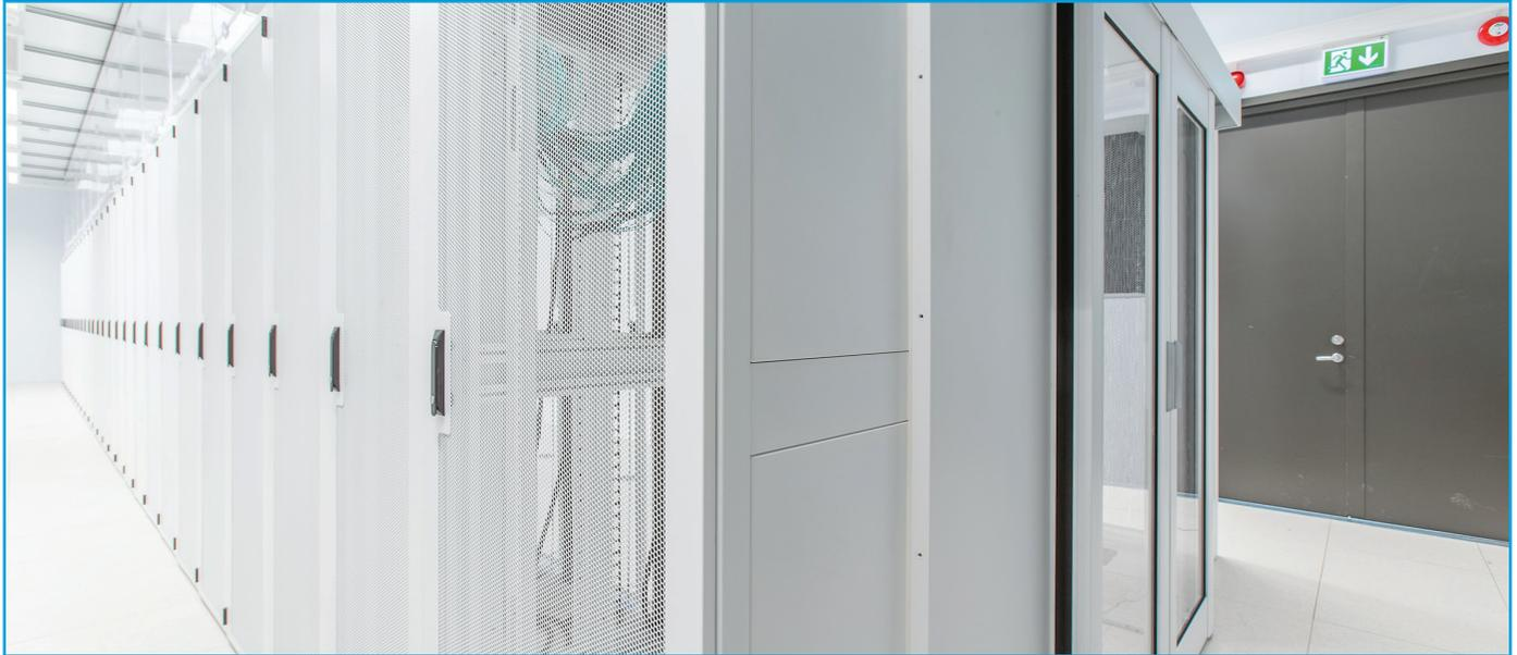
CPI's BTS Kit effectively isolates hot exhaust air and directs it back to the air-to-air cooling system, increasing cooling efficiency.
