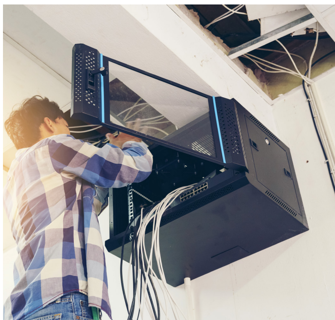
FIGURE 4: Installing cables in a zone enclosure.
